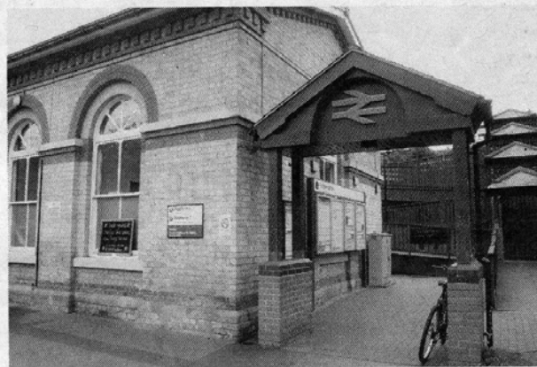
East Midlands Trains have replaced lighting at Lea Road
