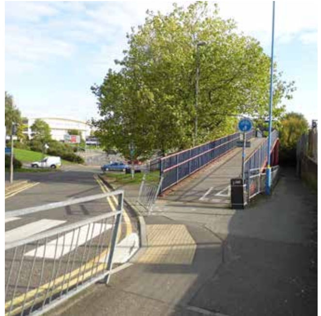
It is not clear that pedestrians need to go under the bridge to find the route to the town centre
